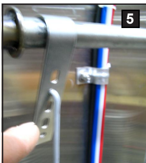
Adjust Door Spring Tension
