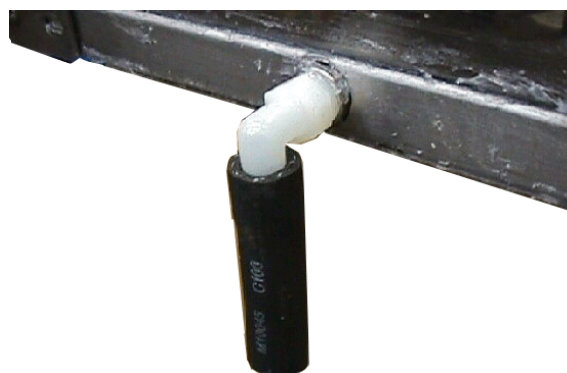
Figure 10 - Install drain fitting on the inter-unit barrier bracket.
