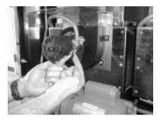
4. Remove wire nuts connecting blower motor wires to wires in conduit.
