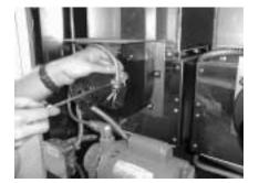
5. Loosen conduit from blower motor.
