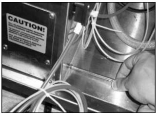
Removing the screws for the electrical box cover.
