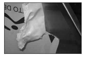
Remove any protective plastic prior to installation.
