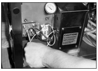
Removing the heater nuts.
