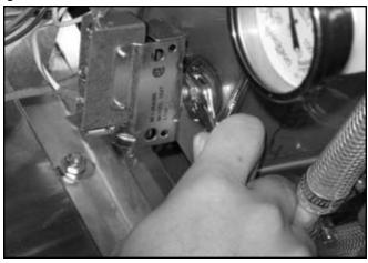
Removing the probe and imperial brass fitting.
