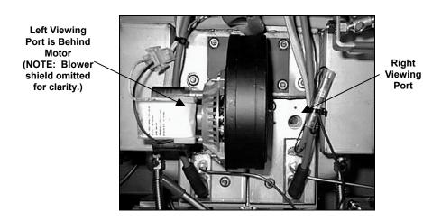
The air/gas mixture is properly adjusted when the burner manifold pressure is in accordance with the applicable table on page 5-8 and the burners display a bright orange-red glow. If a blue flame is observed, or if there are dark spots on a burner face, the air/gas mixture requires adjustment.
