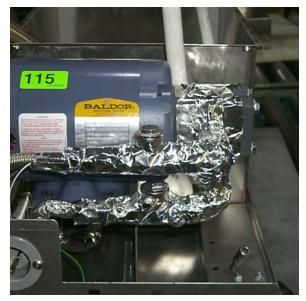
Heater strip installed [115V PF50 (Return/Suction)].
