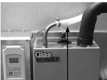
Install and insulate glycol line from heat exchanger to bath
