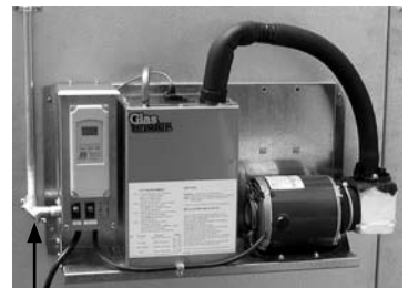
Install power line between condensing unit and control panel.
