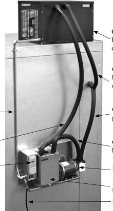
Condensing unit and heat exchanger cabinet
