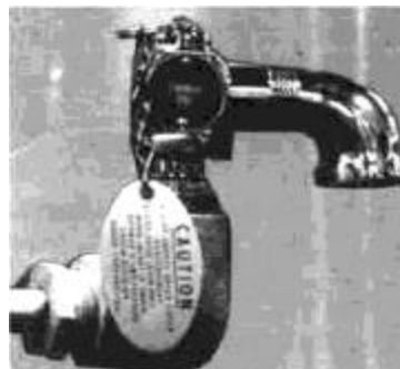
Safety valve with elbow in correct position
