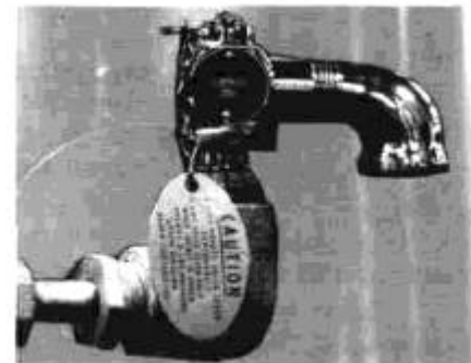
Safety valve with elbow in correct position
