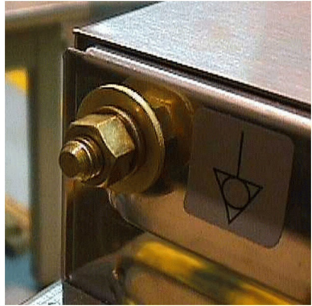
The equipotential terminal is located on the left rear of the units.
