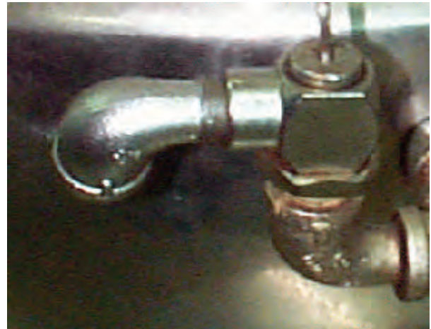
The open end of the pop safety valve elbow must face downward.
