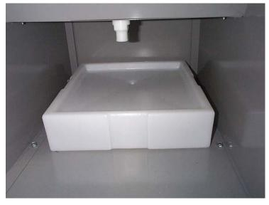
Clean out the lower drain pan. Pour hot water into the drain to be sure that it is clean.
