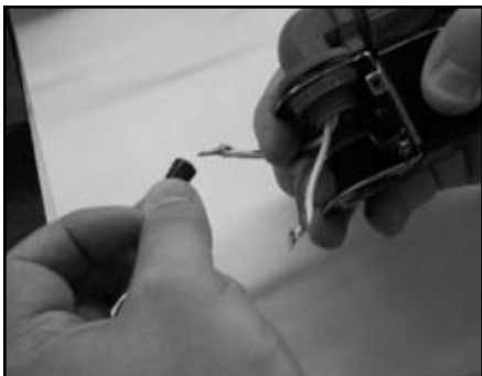
Removing the wire nuts
