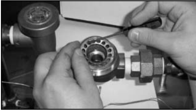
Removing the screen retainer
