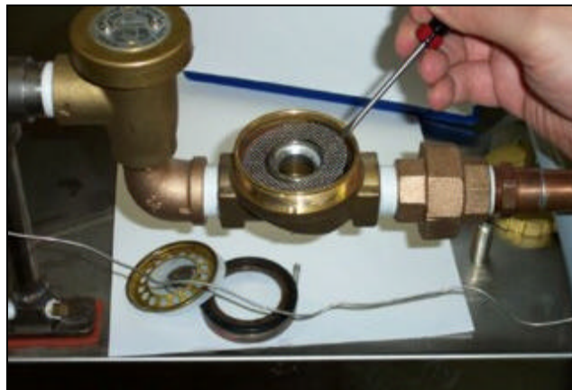
Removing the mesh strainer screen
