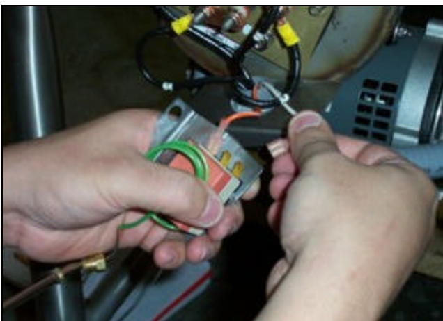
Removing the wires from the thermostat.
