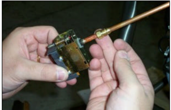
Sliding imperial fitting onto new thermostat.
