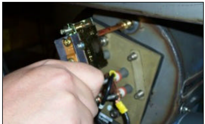
Putting the new thermostat in the well.
