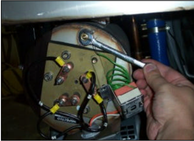
Removing the imperial brass fitting.
