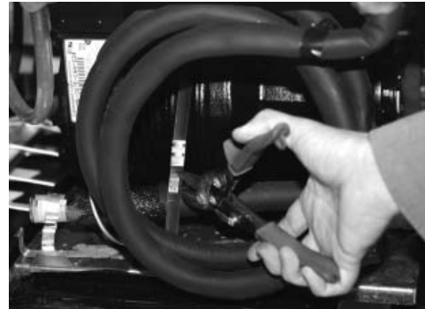
Cutting band that is around compressor
